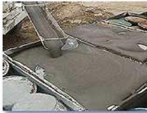
Figure G3-2. Filling voids around drums at EnergySolutions Facility in Utah. Figure taken from EnergySolutions Web site.
