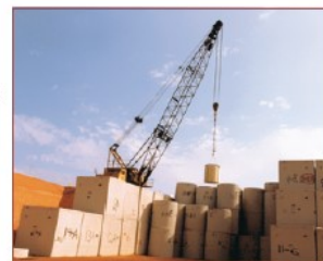
High Integrity Container of Class A LLRW being placed in a cylindrical disposal vault.
