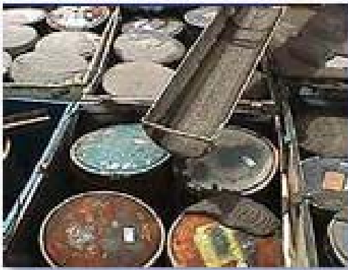
Figure G3-2. Filling voids around drums at EnergySolutions Facility in Utah. Figure taken from EnergySolutions Web site.
