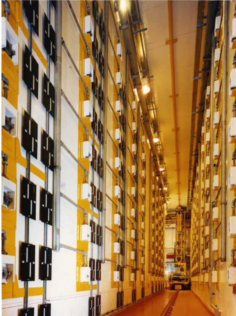
Figure E3-2. Remotely operated store for pure \text{PuO}_2 in welded stainless steel canisters in the THORP facility at Sellafield, U.K.
